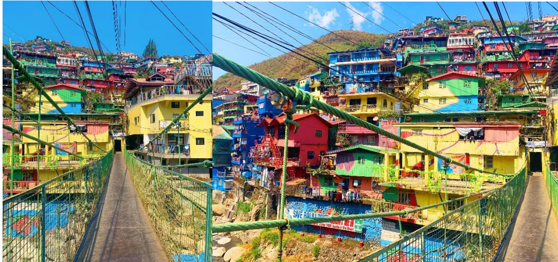
Figure 7: Suspension bridge at village entrance
