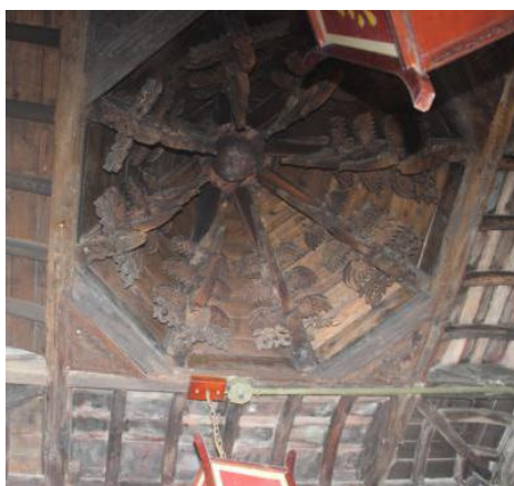
Figure 9. Ceiling of dunxu stage
