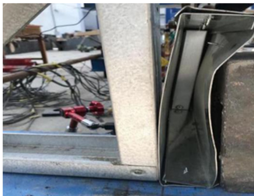
Figure 5. Local buckling failure of box girder
