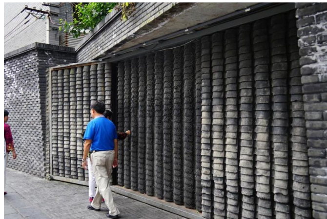
Figure 3. Breathing tile wall
