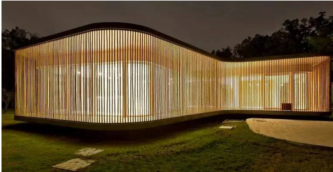
Figure 2. Bamboo for building façade decoration
